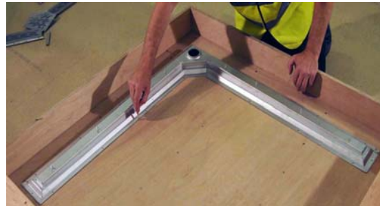
Fig 8. Marking Channel Position in Floor
