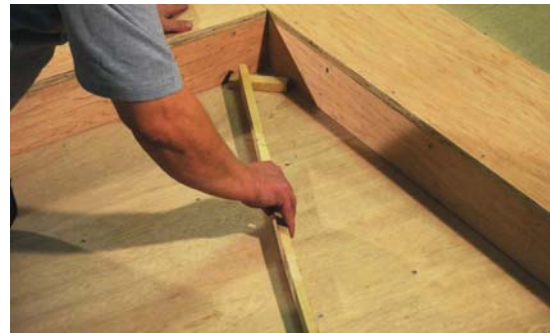
Fig 3. 15mm Batten to Set Fall to Channel
