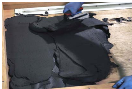
Fig 4. Creating Rough Falls to Channel
