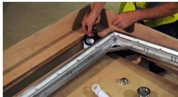
Fig 9. Installation of Trap
