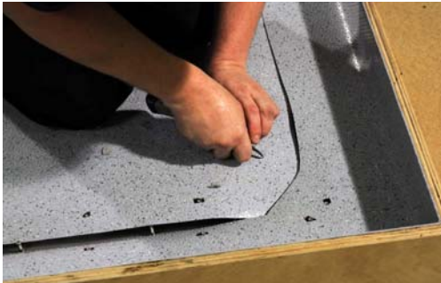
Fig 11. Cutting the Vinyl Into Channel
