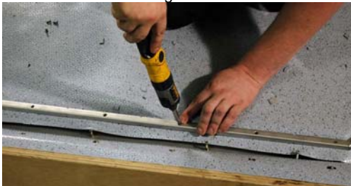
Fig 12a. Dressing Vinyl Into Channel
