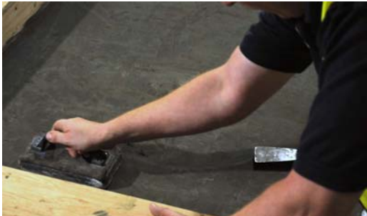
Fig 7. Final Smoothing of Compound
