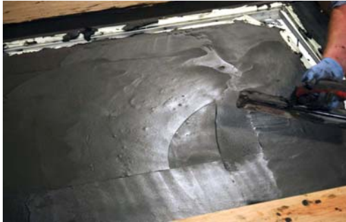
Fig 6. Final Levelling to Falls
